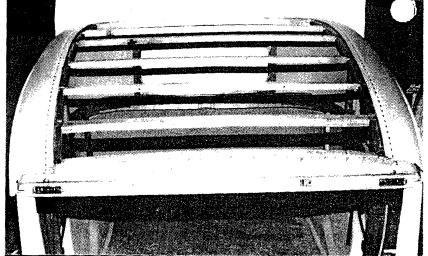
In this photo you will see all of the roof rips in place. Note the two metal inserts in the front header. These are the backing plates for the bracket shown on the left. These metal inserts are tapped for the screws. The way this is all joined makes for a strong joint.
